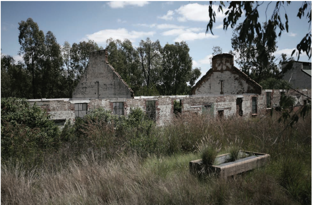
Figure 2.24 Existing compound in ruins (2014)
