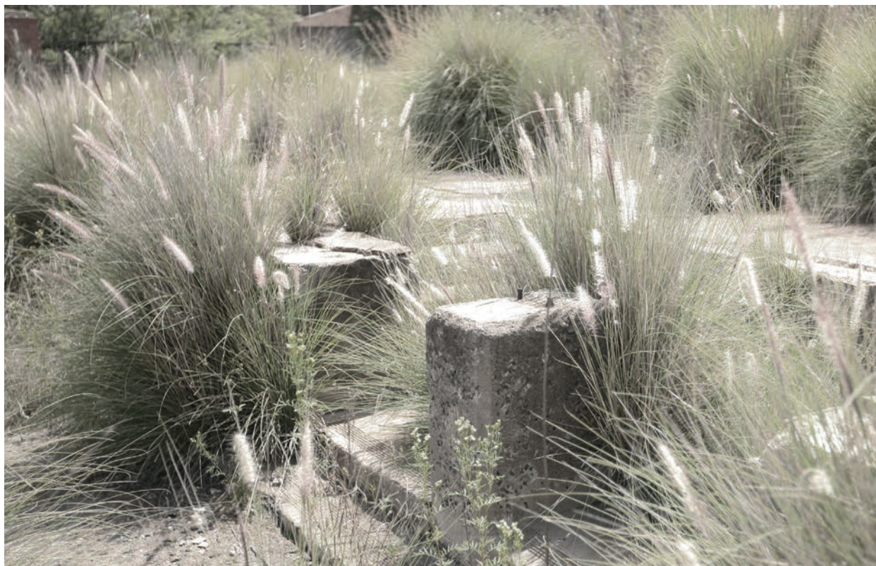
Figure 2.25 Grass growing from existing food preparation and washing square (2014)
