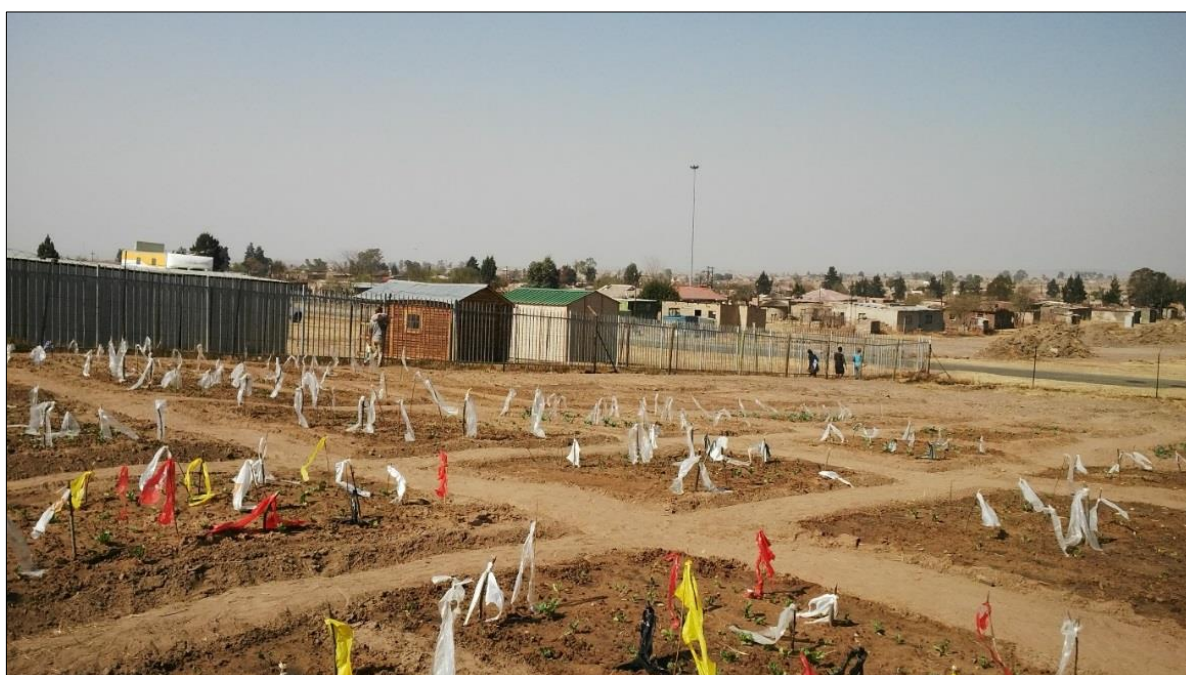
Figure 35 Picture illustrating the progress already made at the Blaauwbosch Primary school
