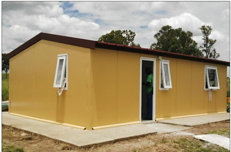
Figure 1B One of the prefabricated houses constructed by ArcelorMittal, for the less fortunate people in their direct communities.
