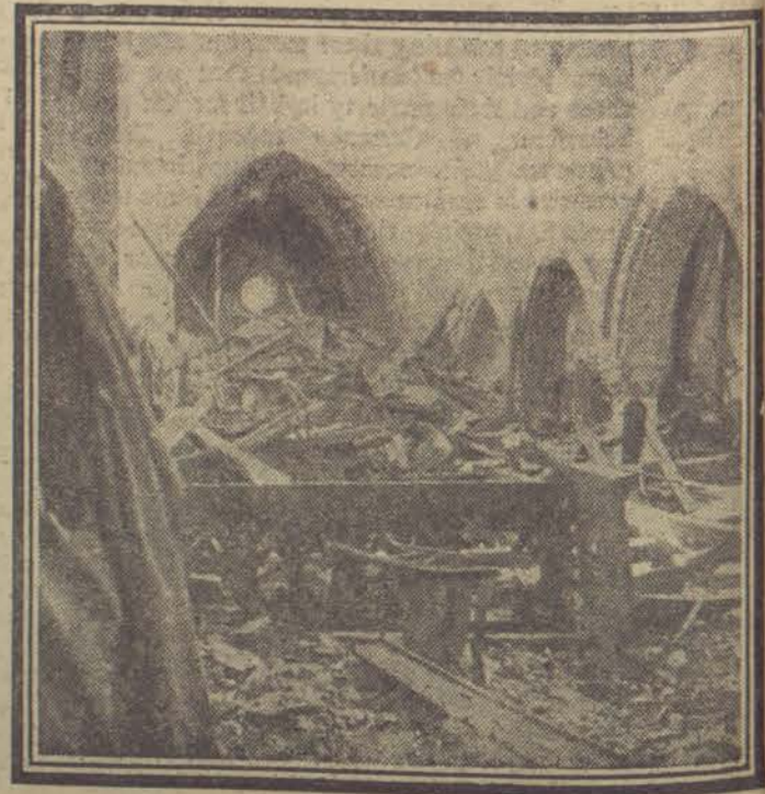
It is war, and the church as well as the brewery is wrecked by the enemy.
