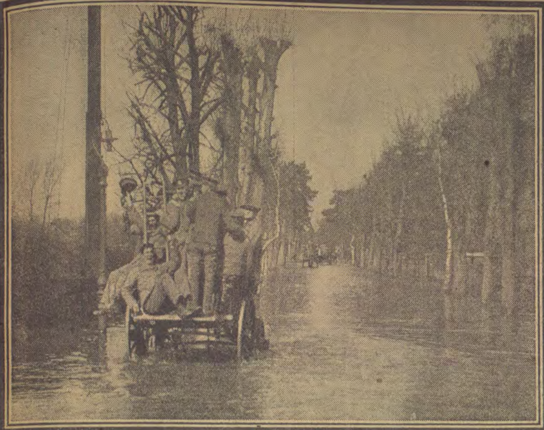
Heavy rains have caused a rapid rise of the Thames, and the roads around Maidenhead are flooded. But this party of Royal Engineers managed to find a way back to camp.
