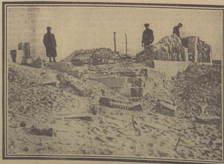
Belgian engineers when blowing up this villa at Coxyde found that its walls were more than a yard thick, and gun platforms of concrete had been laid.
