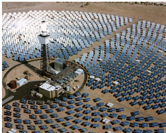
Figure 1.1 Solar One, Barstow, California [3]
