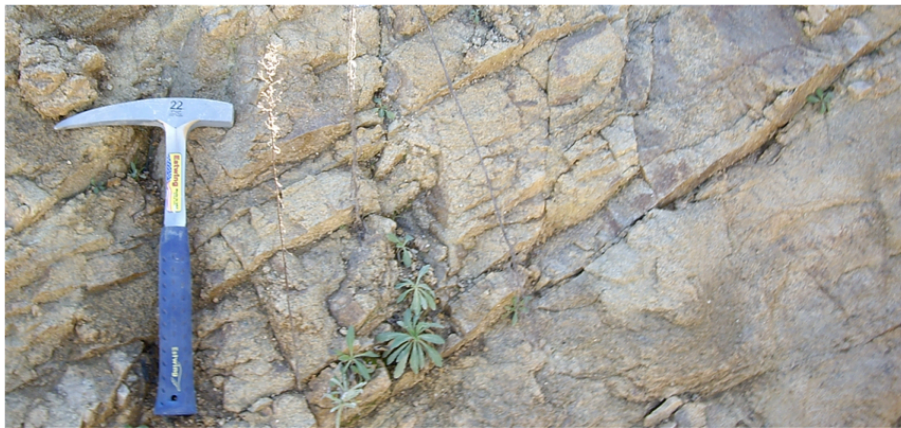
Figure 2-7. Secondary porosity in the form of parallel joints in fractured Lanseria Gneiss (Johannesburg Dome Granite) from Midrand (Gauteng Province, South Africa); note the varying apertures.
