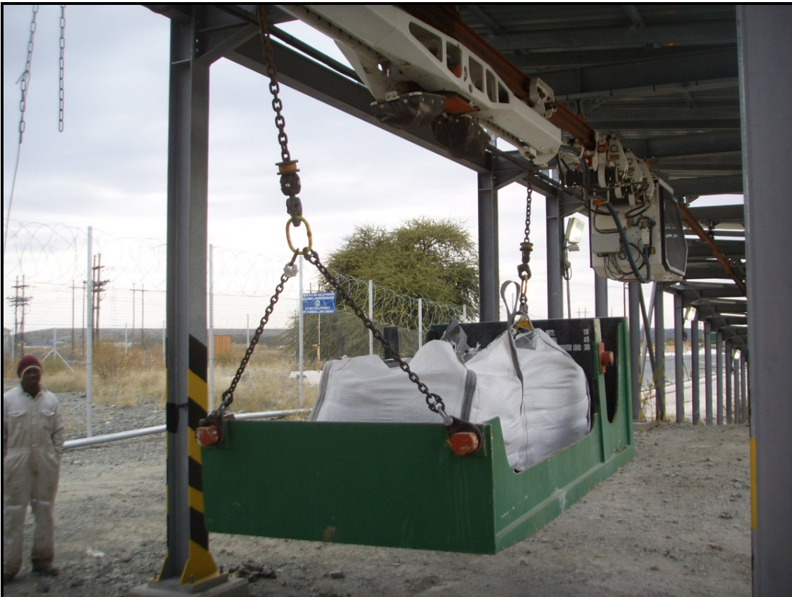
Figure 2.7b: Monorail Transportation System Infrastructure (Material cassettes) (AAP Union Section Mine, 2008)
