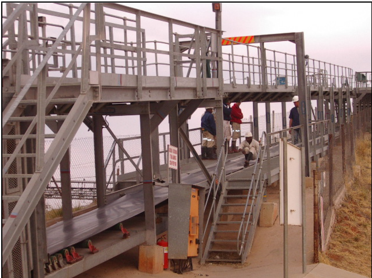
Figure 1.4.3: Surface conveyor belt training at North Shaft (BRPM, 2008)
