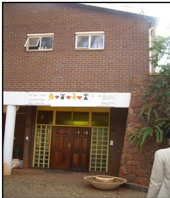
Figure 3.1: Main entrance of the residential care facility
