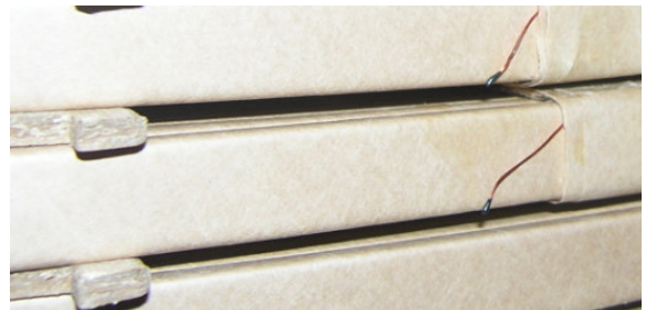
Figure 15 Thermistors mounted at the oil outlet of a full size winding.
