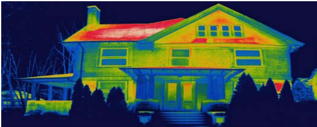
Figure 9 : Thermal survey of a residential property
