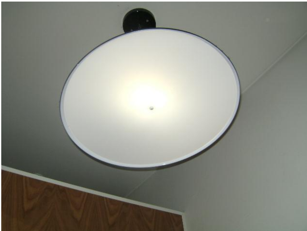
PHOTO 10: LIGHTING IN BROOKLYN (P2:13)
