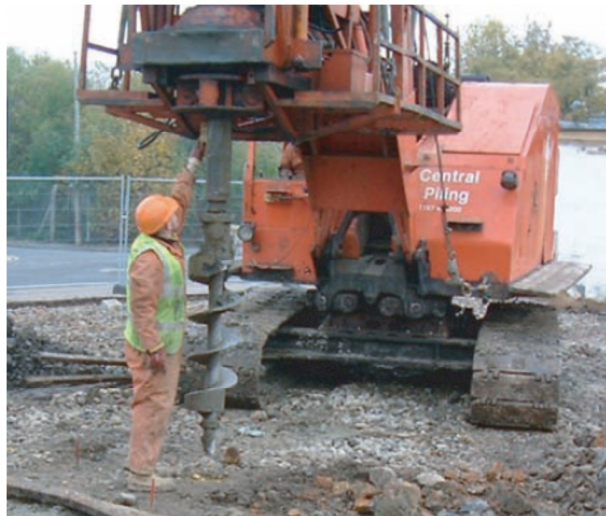
Figure 15: A piling rig ( http://www.bne.uwe.ac.uk )
