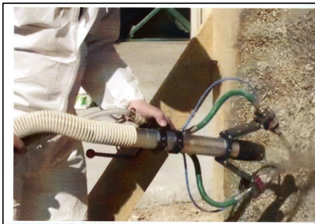
Figure 2 Spray on application of hempcrete (Allin, 2012)
