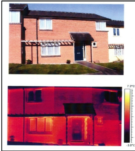
Figure 6 Thermographic image of house constructed using masonry (Allin, 2012)
