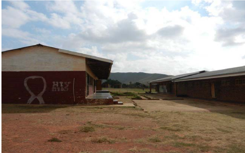
Photograph 1.2: Rural primary school (School 3)
