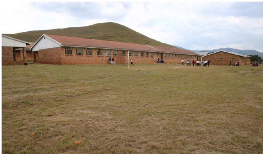
Photograph 1.1: Rural secondary school (School 1)
