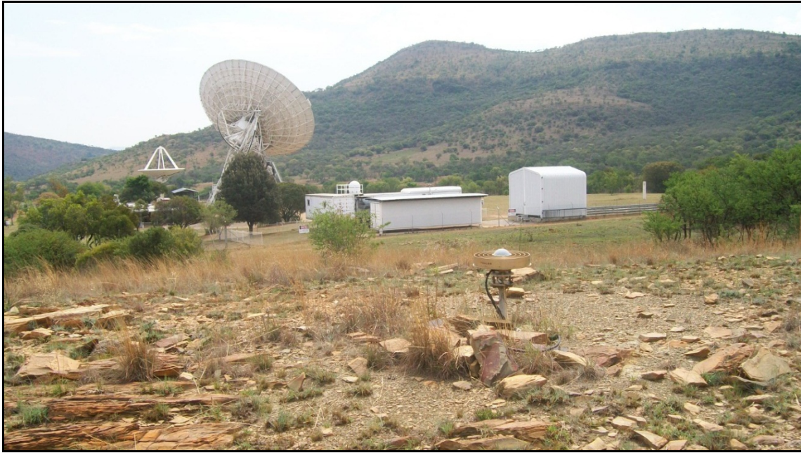
Figure 1. Geodetic instruments collocated at HartRAO, South Africa. In the far distance left, the 15 m VLBI antenna, left-foreground the 26 m VLBI antenna, centre-foreground the SLR (MOBLAS-6) station, right-centre the Lunar Laser Ranging (LLR) in development and the IGS GNSS station (HRAO) antenna in the foreground.
