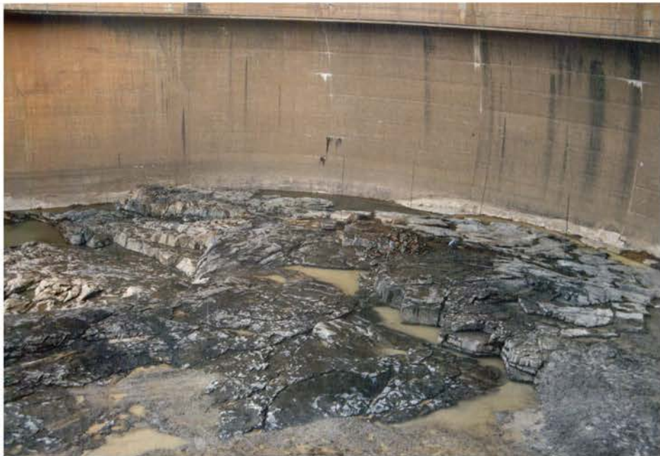
Plate 20 Jointed dolerite downstream of the left downstream area (Van Schalkwyk).
