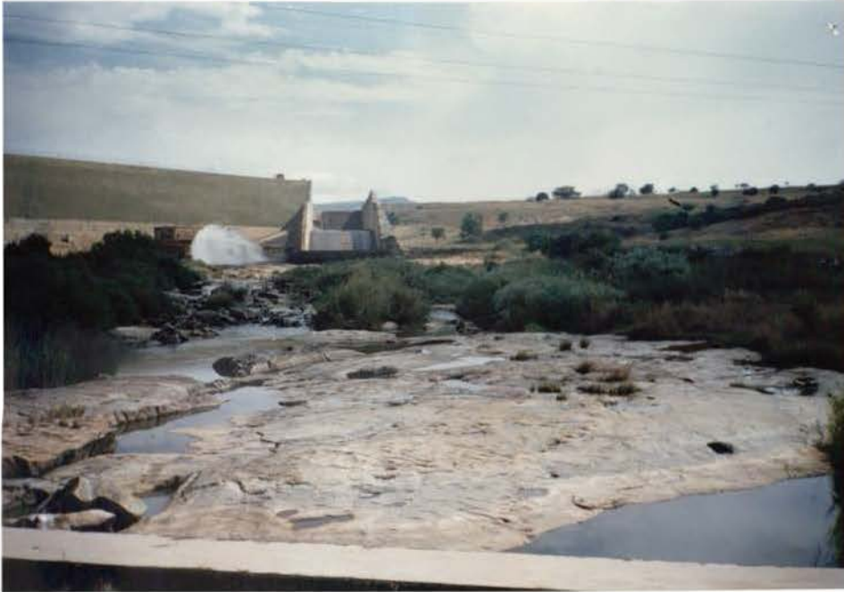
Plate 29 Vygeboom Dam - Partially lined, side-channel spillway with flip bucket.
