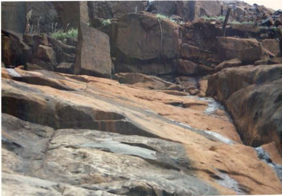
Plate 23 Depth of erosion from the original ground depth, on the left downstream area of the arch.
