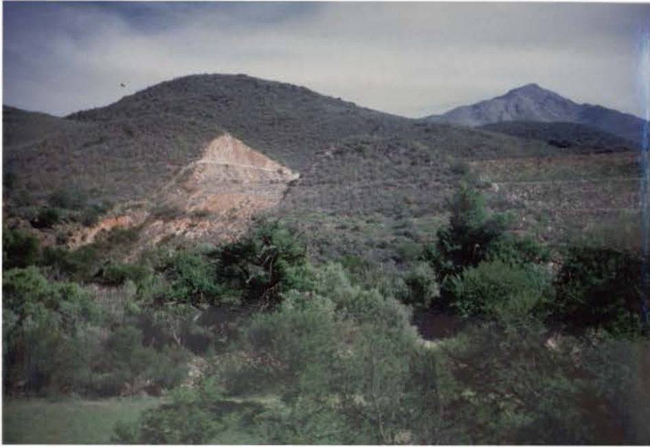
Plate 4 Koos Raubenheimer Dam - unlined side channel spillway.
