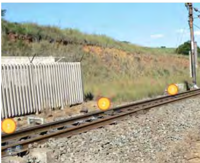
Figure 5: Bloubank test site (Coal Line) with three test stations
