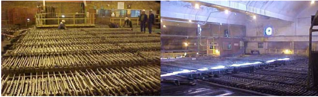
Fig. 5 Cell house working surfaces
