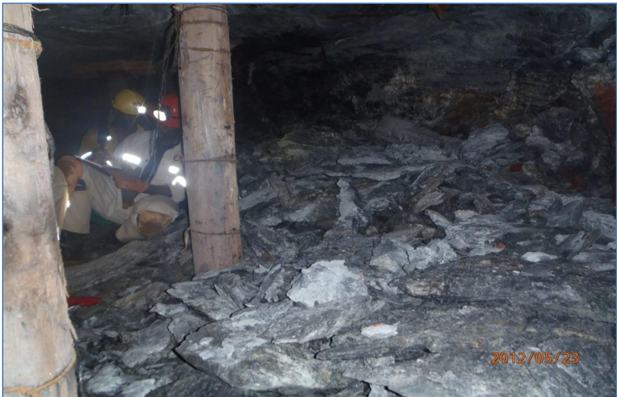
Figure 30: Damage caused by a face burst
