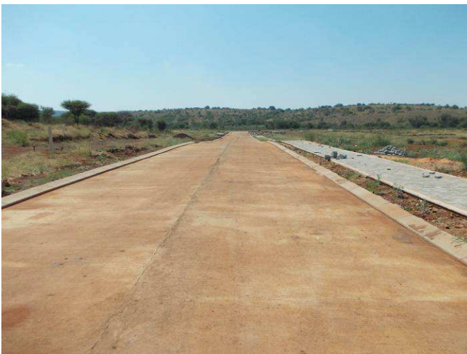
Figure 10: Completed UTRCP with Kerb and Sidewalk.
