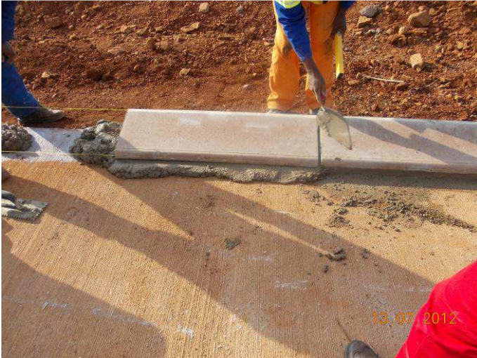
Figure 9: Kerb constructed on UTRCP.
