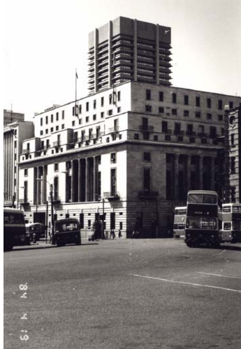
Figure 5. Digitized from the original: photograph taken on 19 April 1984 of the Barclays Bank Building designed by Gordon Leith in 1939 that was digitized from the original
