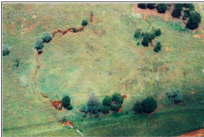
Plate 25. Subsidence in Bapsfontein, Ekurhuleni (2004), due to dewatering (Photo taken from Wagener, 2008).
