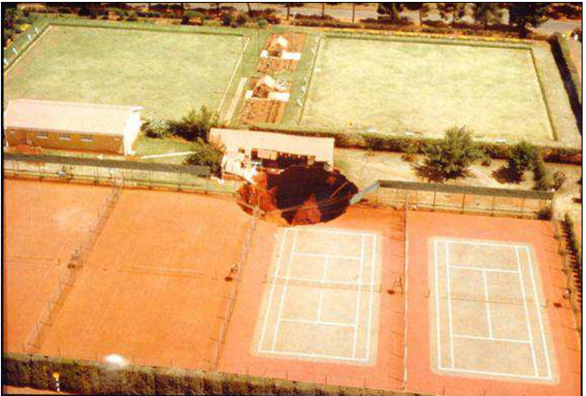
Plate 31. A sinkhole at Venterspost recreational center that swallowed part of the club house and one spectator on 24 October 1970 ( Picture from CGS files ).
