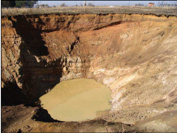
Plate 15. Sinkhole in Bapsfontein, Ekurhuleni (2004), as a result of dewatering. (Photo by A.C. Oosthuizen, CGS).
