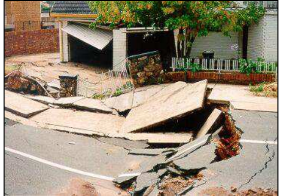
Plate 8a & b (view towards house): Sinkhole at house in Centurion, due to a leaking service (Photos from CGS archives, referenced by Waltham et al., 2005 as taken by/from F. Bell).
