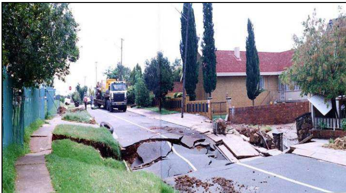
Plate 8a & b (view towards house): Sinkhole at house in Centurion, due to a leaking service (Photos from CGS archives, referenced by Waltham et al., 2005 as taken by/from F. Bell).
