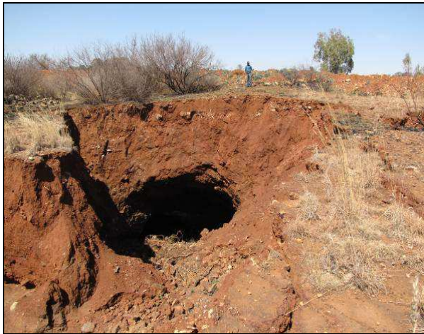
Plate 17. Sinkhole near Carletonville, West Rand (2010), due to a leaking and overflowing canal. (Photo by S.Richardson)
