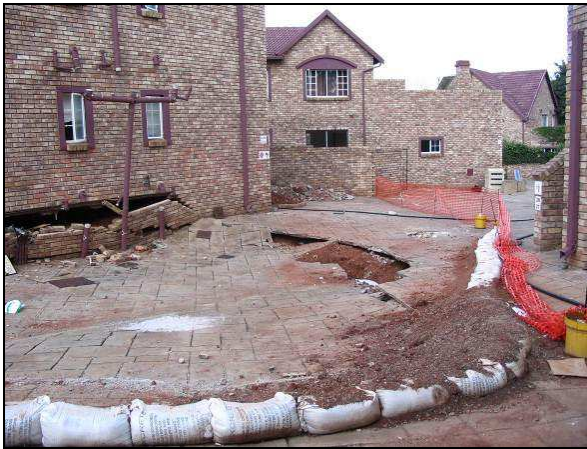
Plate 21. Subsidence in Lyttelton, Tshwane (2008), due to a leaking service (Photo by A.C.Oosthuizen, CGS).
