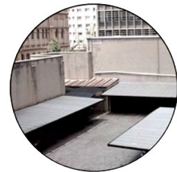
4. Parking structures looking towards theatre lobby
