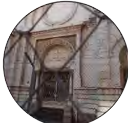
1. Old Synagogue, PTA Highly significant to national heritage as it housed significant trials of struggle heroes such as Nelson Mandela. Abandoned and inaccessible to the public.
