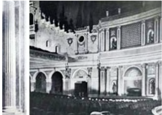
Fig. 3.7.4 Theatre interior 1931- Auditorium (Cinema Souvenirs 2013)
