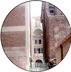
4. View through alley to post office entrance
