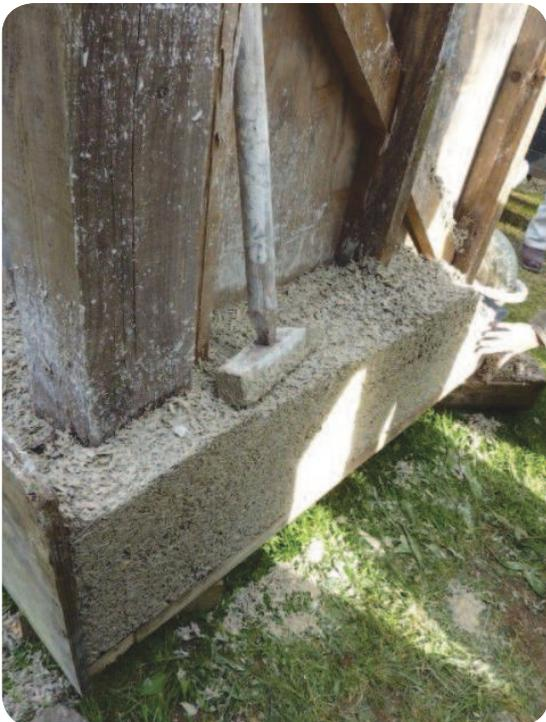
figure\_03.09\_\_wall construction of hempcrete wall, The Hemp House, Noordhoek, Cape Town.
