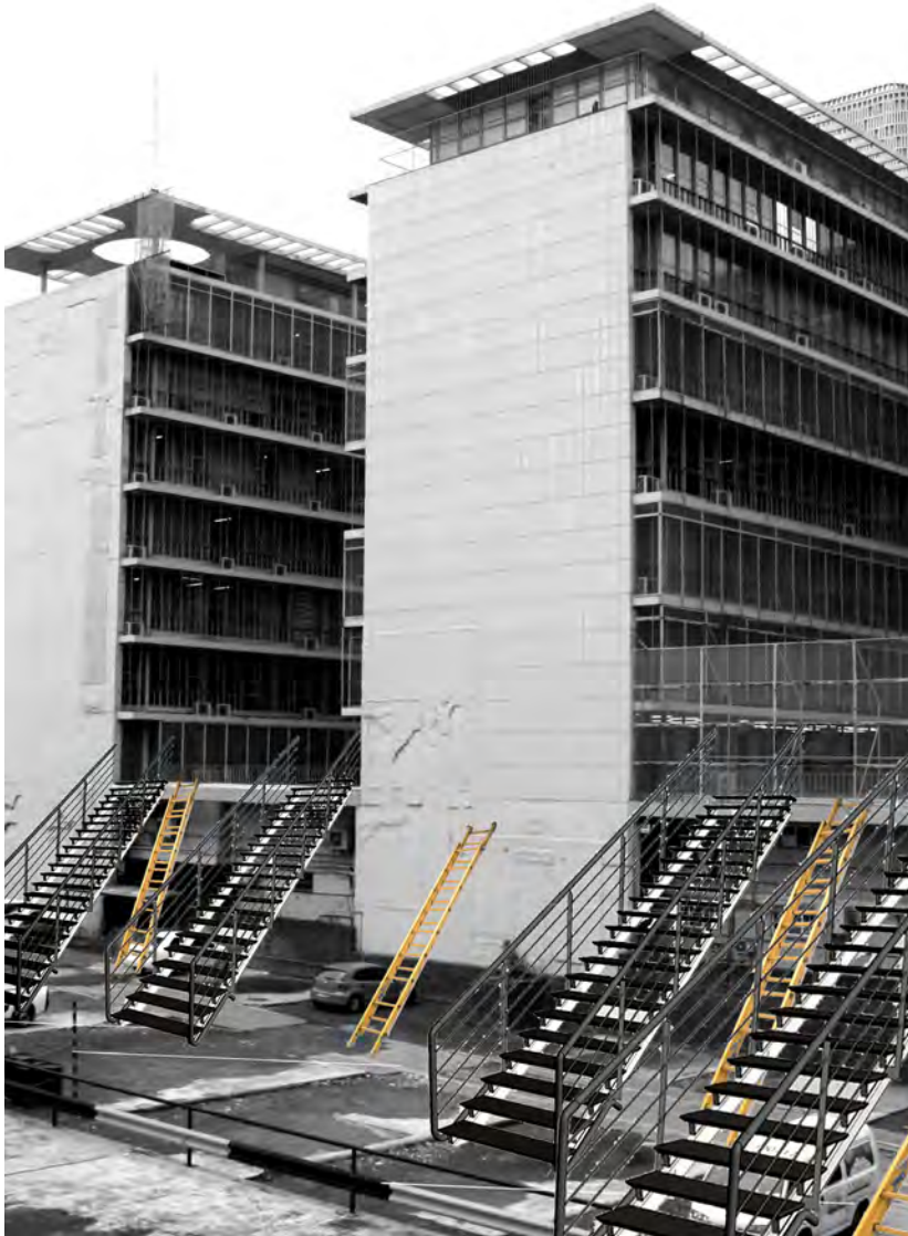
Figure 3_3 - Level as Fence re-imagined on site (Source: Author, 2013)
