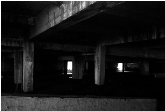
Figure 8_8 - Existing basement structure (Source: Author. 2013)
