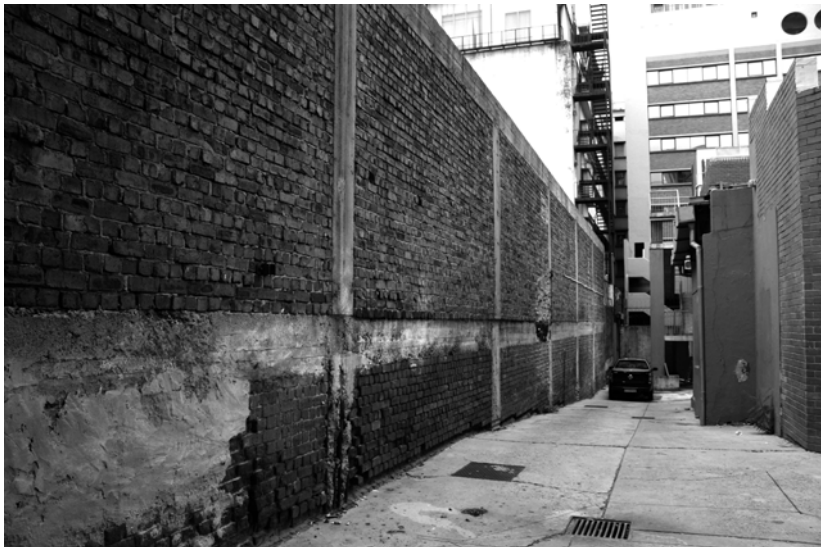
Figure 3_20 - Service Yard from Schoeman Street Entrance (Source: Author, 2013)
