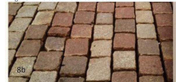
Figure. 7.11 Cobblestone paving
