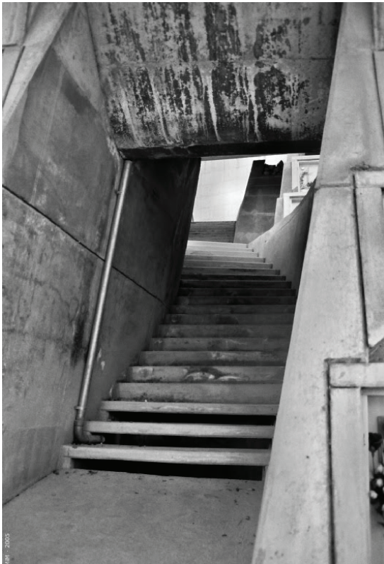
Figure 6.3: Iguualada Cemetery entrance, a physical transition through the quarry by MALLOL & MORETTI, 2005 (FLICKR 2013)
