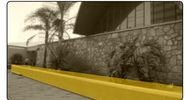
Fig:7.4 Current condition of the pond on the Northern facade
