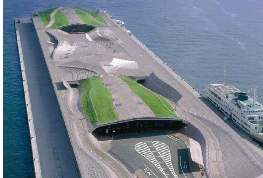
fig 6.7 Yokohama international terminal, Foreign Office Architects (FOA, nd)
