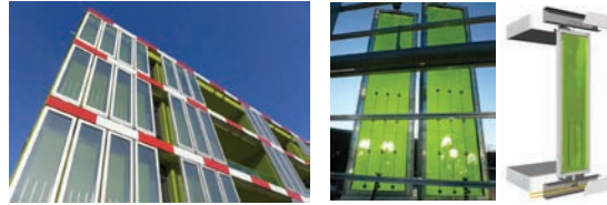
FLAT PANEL PHOTO BIOREACTOR FACADE, BIO HOUSE, HAMBURG GERMANY
