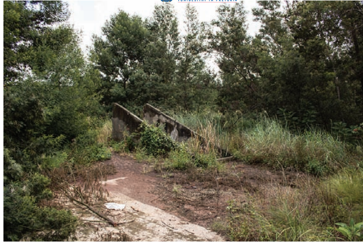
CONCRETE STRUCTURE IN CLAY SOIL
