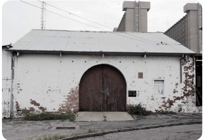
Figure 3.26(c): [iii] Plumbing Store. (Photo by: Philip Slabbert)
