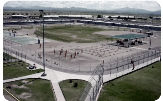
Figure 2.5(b): Arizona State Prison Complex, Arizona.
