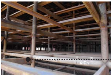
..... Steel channels, sections: beams and columns
