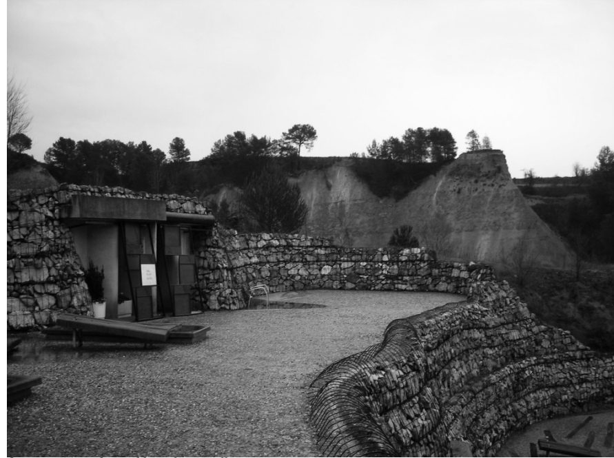
fig. 5.4 _Tiers formed by gabion walls
