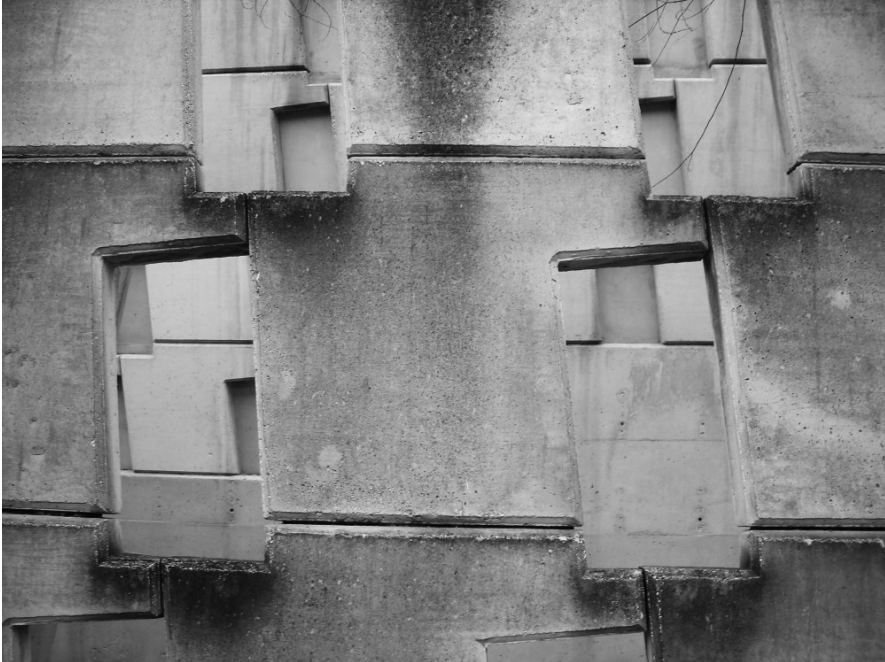
fig. 5.5 _Pre-cast concrete elements
