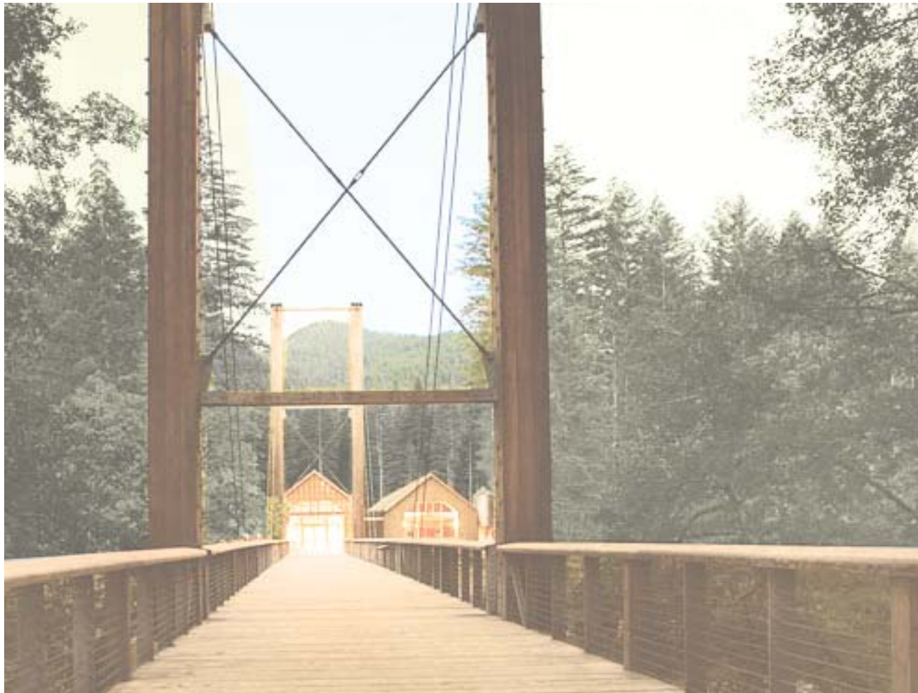
Fig. 8.3: Entrance walkway from bridge (online source: http://www.tillamookforestcenter.com/resources/rental_packet.pdf&h=465&w=310&sz=221&fbid=dl7V_KkALEAIMM&fbnh=275&fbnw=183&zoom=1&usg=__BzgNzaXWNPdcrGZ0pka8fxsgJt0= )
