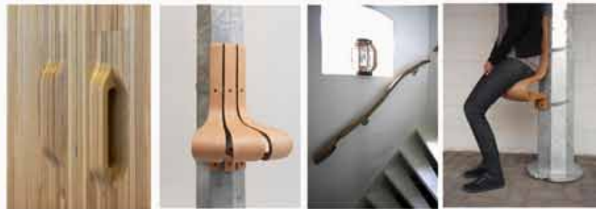
Figure 6-30 Handrails that provide a temporary leaning space
