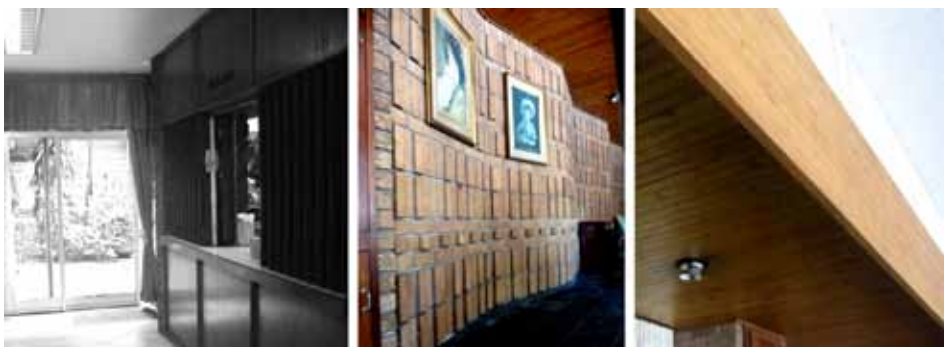
Figure 2-33 Pretoria regionalist characteristics interior shop fitting. Timber boxes constructed in between the columns.
