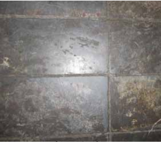
Figure 7-24 Kept slate floors (Author,2013)
