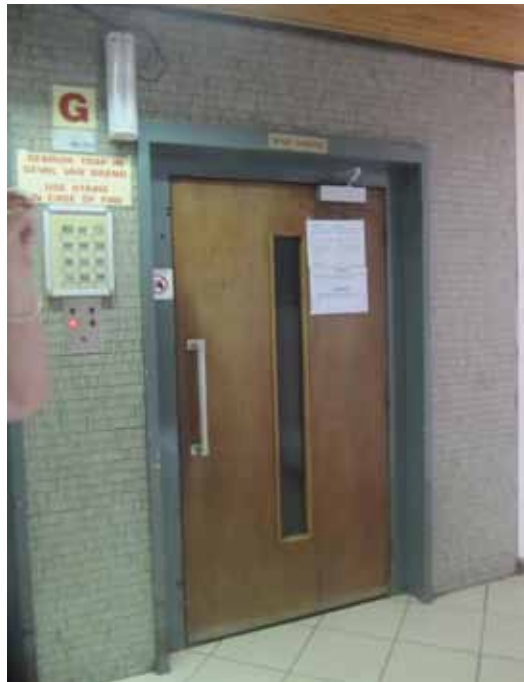
Figure 7-33 Removed lift (Author,2013)
