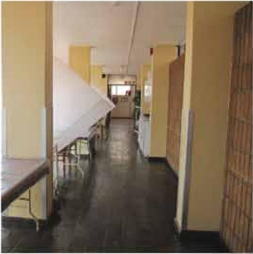
Figure 6-36 Existing passage way
