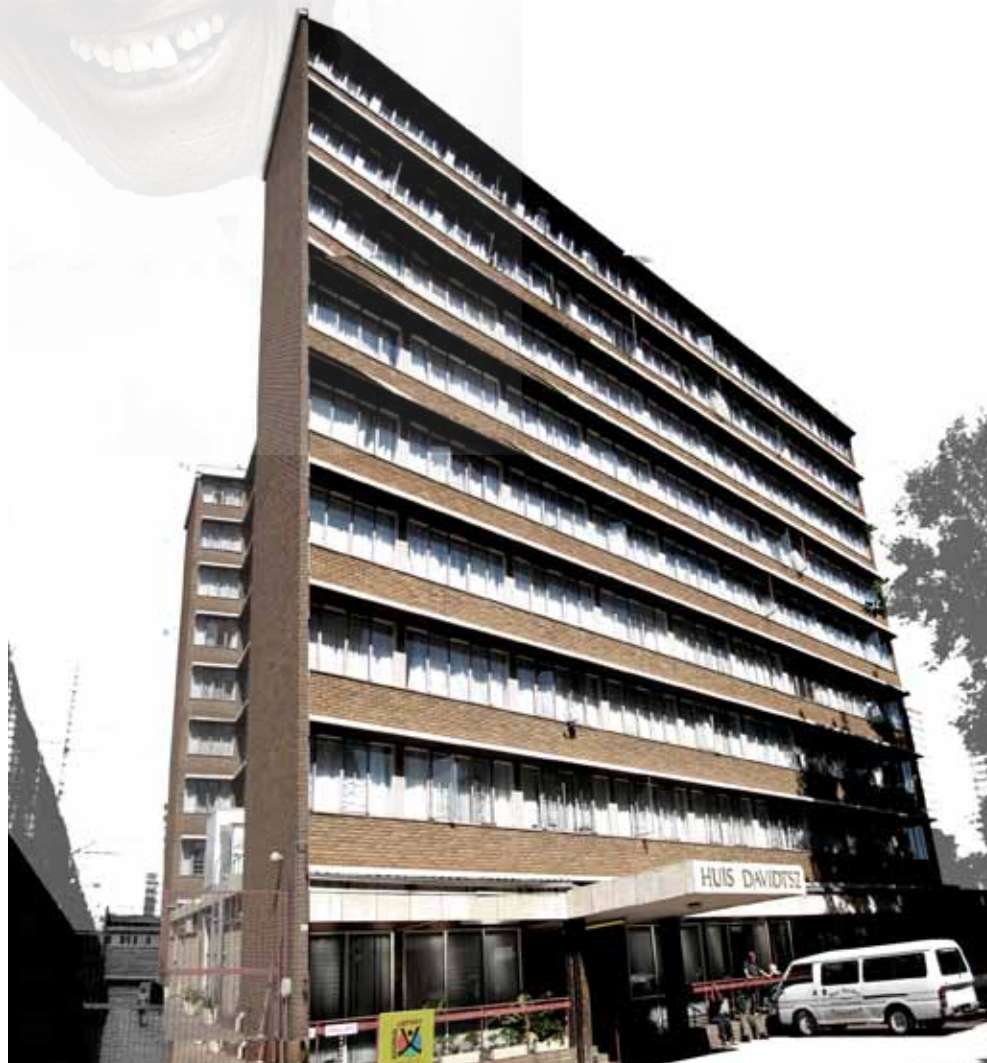
Figure1_21 Northern Facade of Huis Davidtsz
