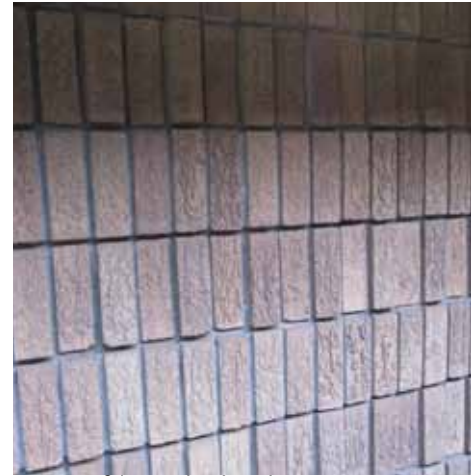
Figure 7-26 Kept brickwork (Author,2013)
