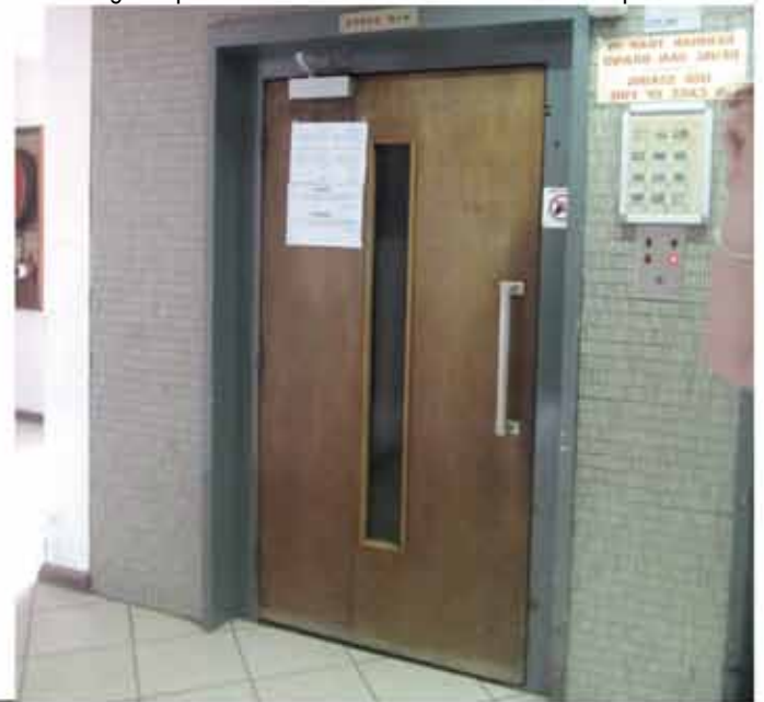
Figure 2-41 Elevator which is the primary form of vertical circulation
