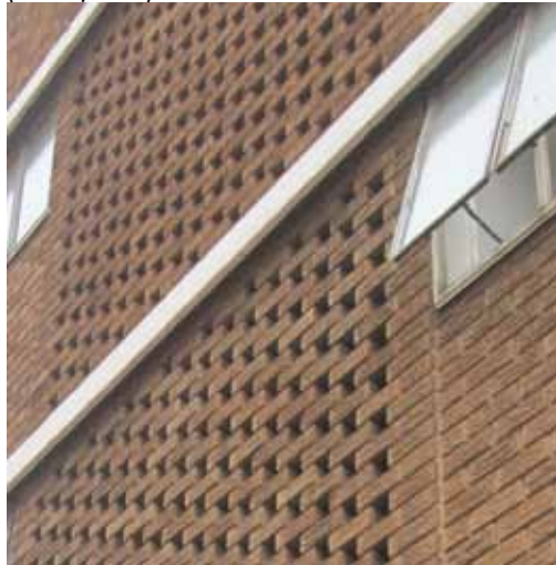
Figure 7-28 Kept brickwork (Author,2013)
