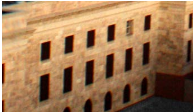
Figure 03.15 Magistrates Court Western Facade
