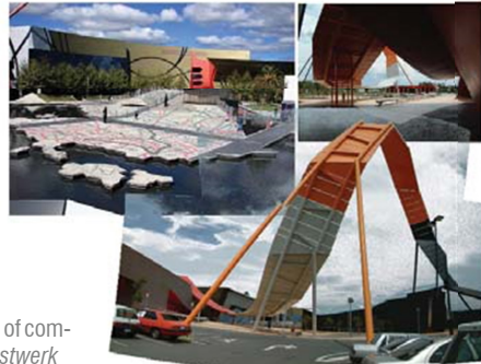
Figure 66: Expressive entrance route canopy known as 'The Uluru Axis' due to its alignment with the Uluru Rock national landmark [Author, 2003]
