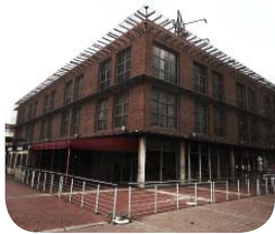
[8] No. 1 Central Place | 2005 |
