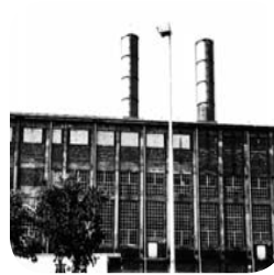
[1] Turbine Hall | 1927 | - Neighbour to Site
