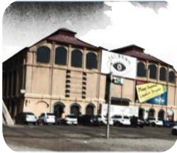
[3] Sci-Bono Discovery Centre in The Electric Workshop [First President Street Power Station] | 1906 | - Distant Neighbour to Site
