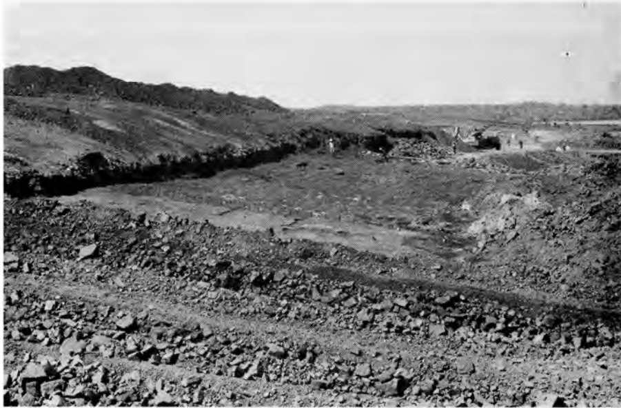
Fig. 19. One of the quarries on the Main Magnetitite Seam at the Mapochs Mine, Roossenekal.
