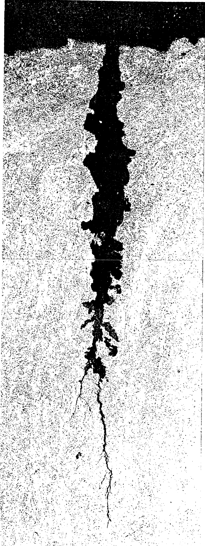
FIGURE 39 A cross-section through cracks found in welds in the high pressure lean gas system at the operating plant. The cracks are wide at the top due to corrosion but are sharp and branched at the base, typical of SCC.
