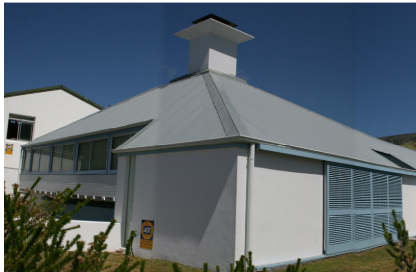
4. View from the south-east corner
