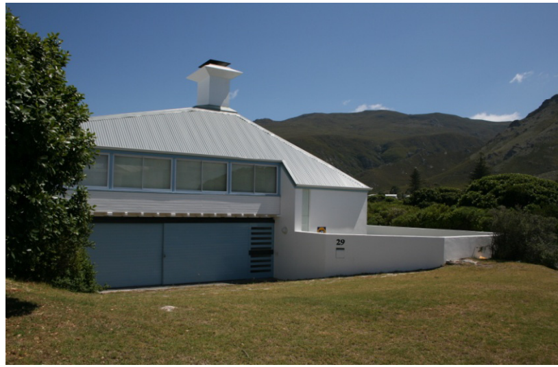
1. View from the south
