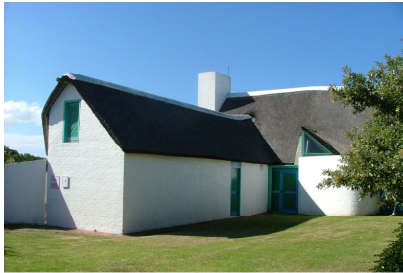
2. View looking north-east
