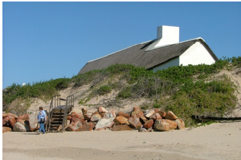
4. View from the beach looking south-west
