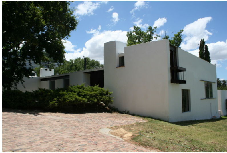
2. View of the south-west corner
