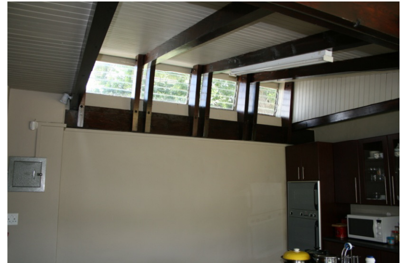
6. Detail of the kitchen roof light
