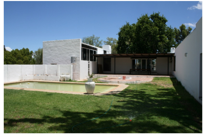
3. View from the courtyard looking west
