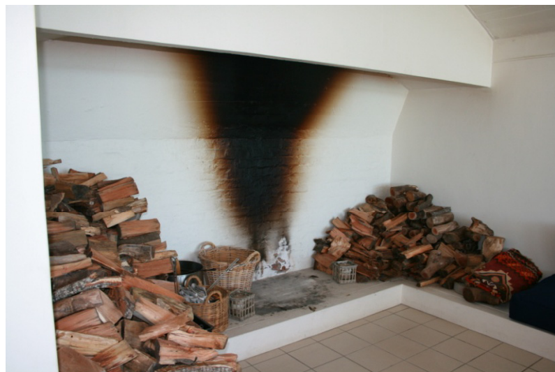
7. View of the fireplace
