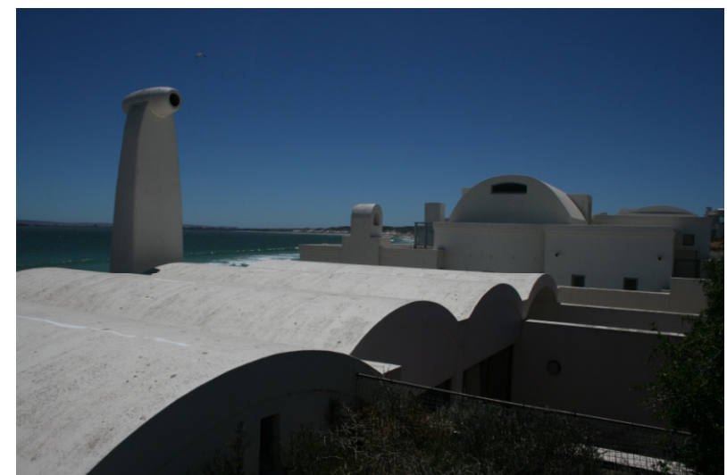
10. View of the roof looking north-west
