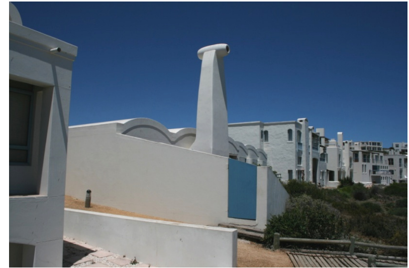
3. View of the north-west corner
