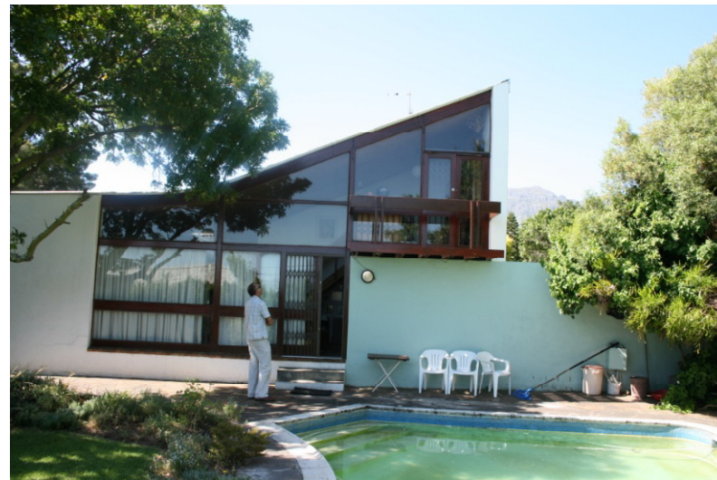
5. View of the south-western facade
