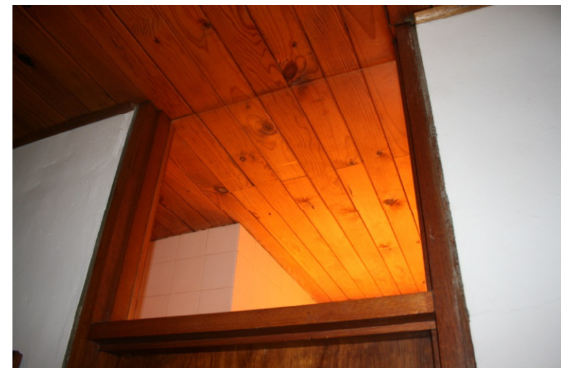
10. View of the door head meeting the roof
