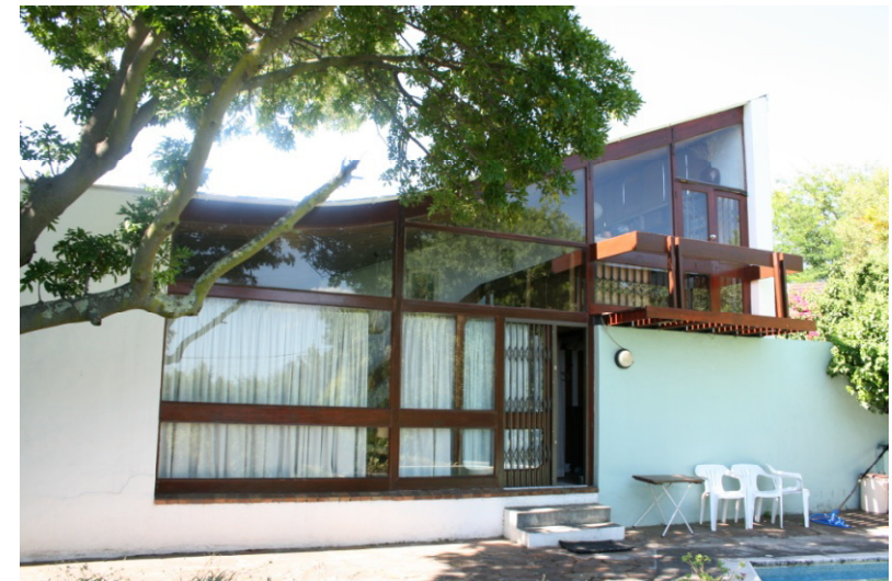
6. View from the garden looking east
