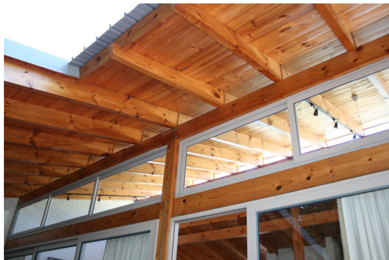
7. Detail of windows above the eaves
