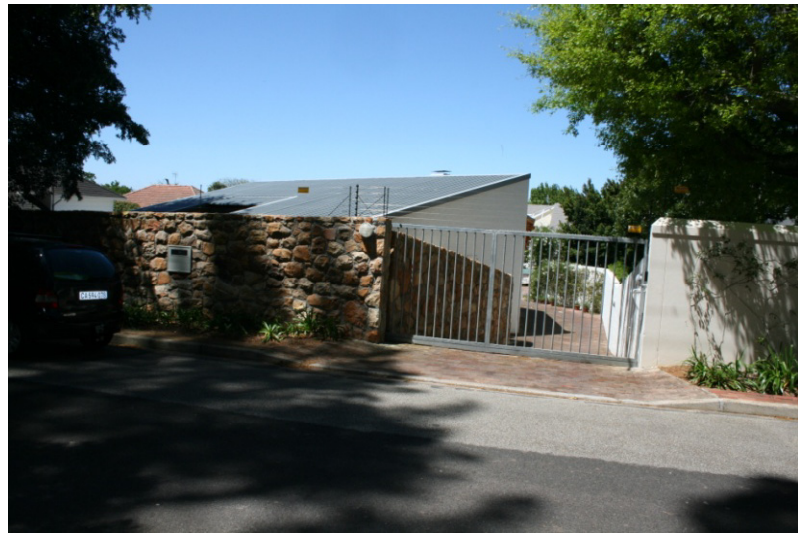
1. View from the street looking south-east
