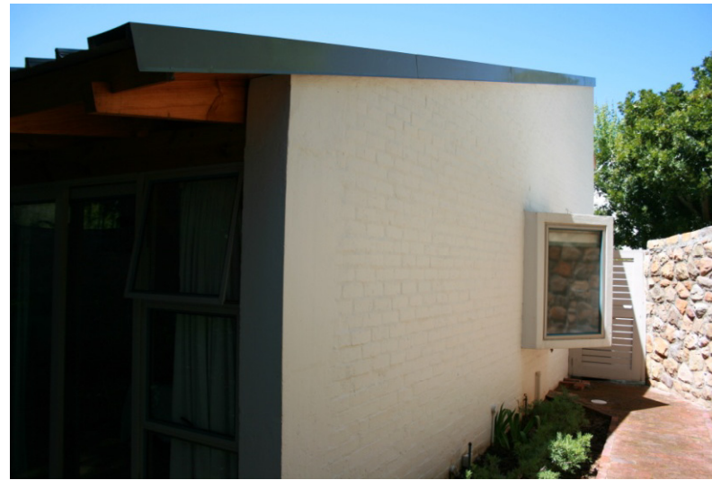
2. View of the north-west corner
