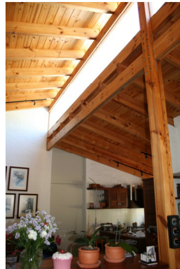
8. Detail of clerestory
