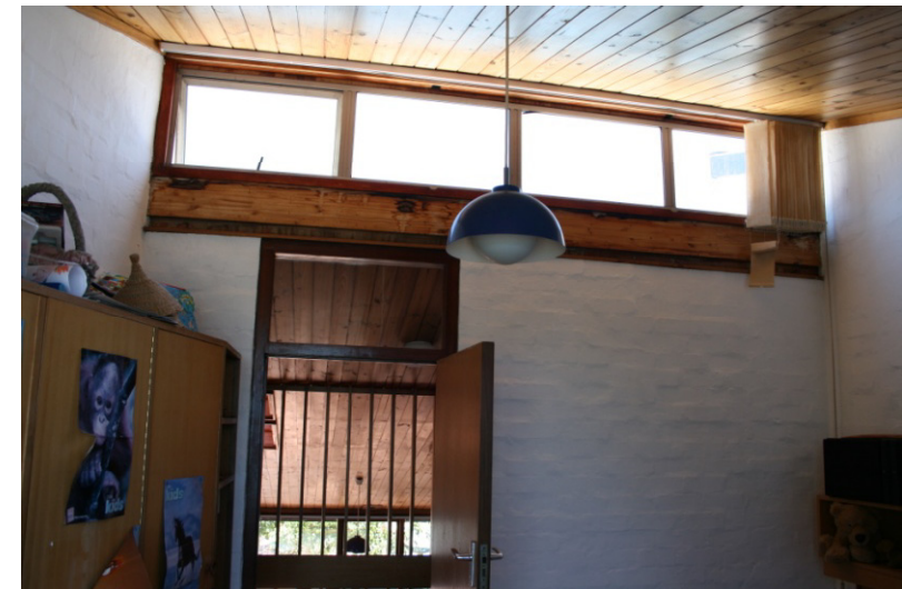
6. View of bedroom clerestory window
