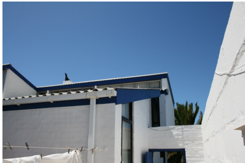
4. View of the west corner
