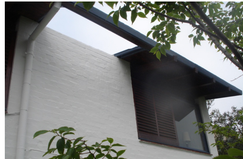
10. View showing wall and roof junction
