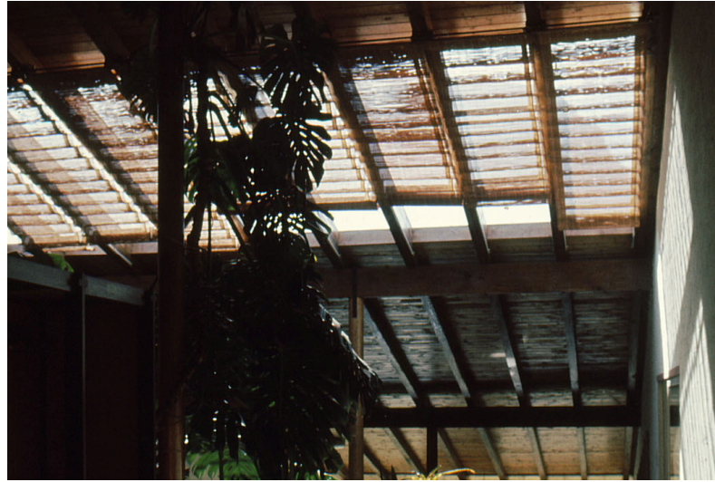
5. View of atrium roof
