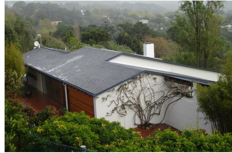
3. View of the garage and entrance looking west
