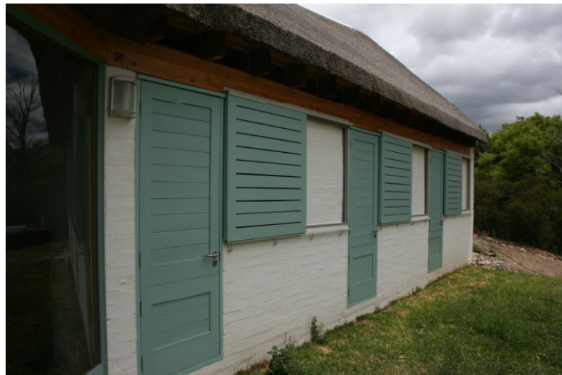
4. View of bedrooms exterior wall
