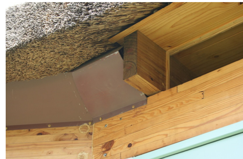
10. View showing junction of eaves treatment and clerestory window
