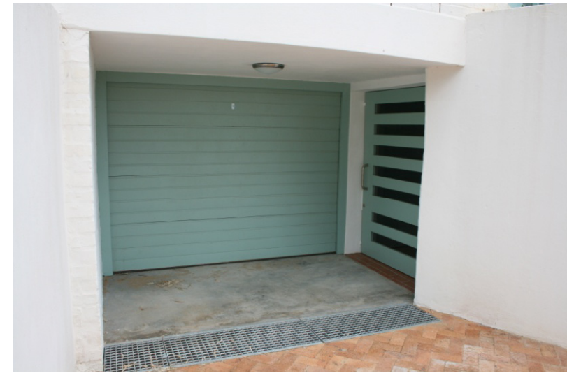
3. View of the garage and entrance
