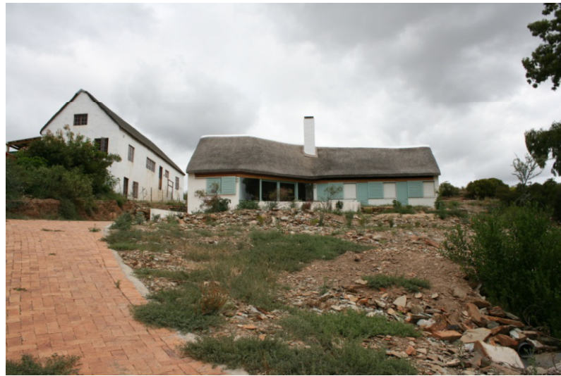
1. View from the driveway looking south-west
