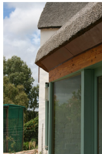
8. View of eaves detail
