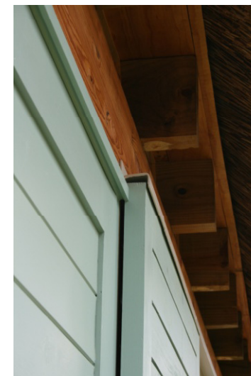
9. View of eaves detail
