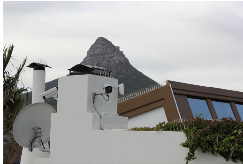
2. View of the roof from the street
