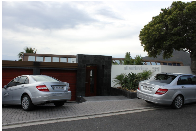
4. View from the street looking north-west
