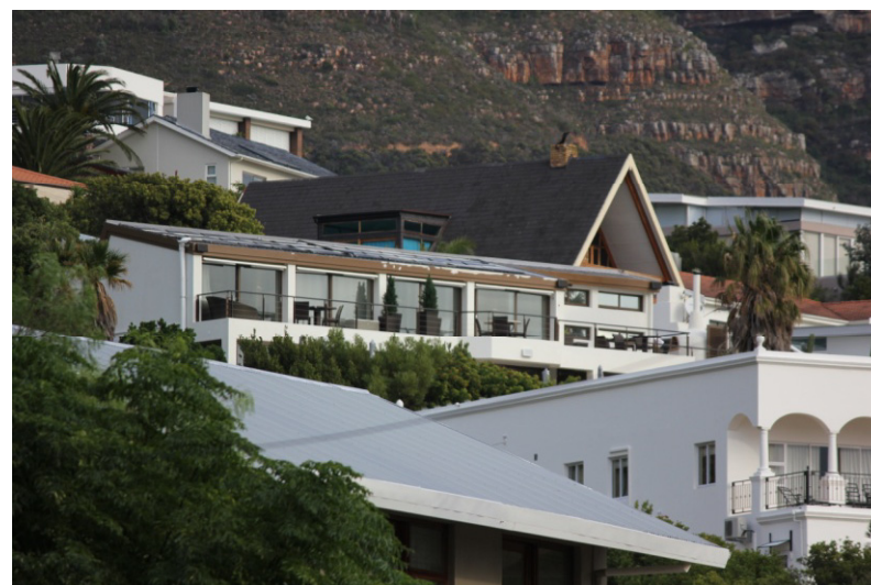
8. View of north-western facade
