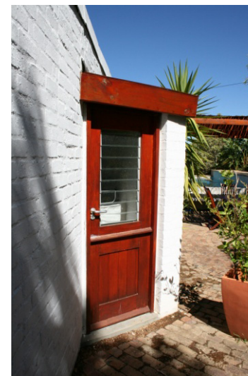
9. Detail of door on northern facade
